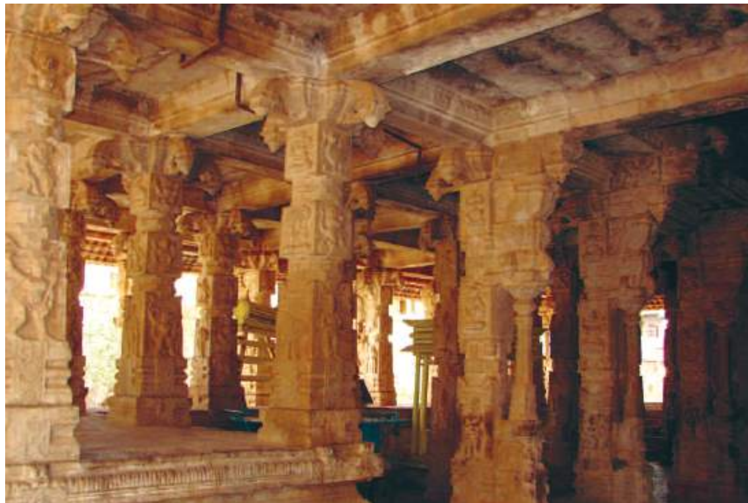
Main Mantapa of the Somesvara temple in Kurudumale, Kolar district. Photo by Hariharan Arunachalam
